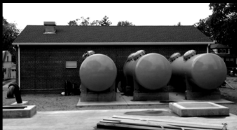
Iron Removal Plant at Well Station No. 28 nears completion
